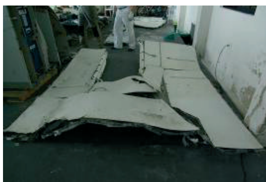
Ceiling of the LDMCR: with top-downwards deformation
