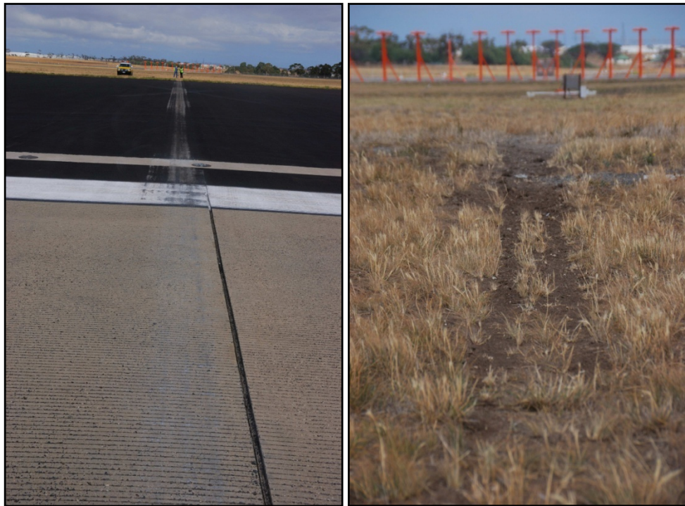
Figure 9: Typical contact marks on runway, stopway and grassed areas
