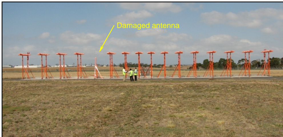
Figure 12: Localiser antenna array
